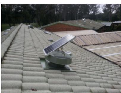
Whirlybird Installation – is very similar to installing a Solar Whiz – and many of our dealers actually prefer to install the Solar Whiz – as it, **unlike the “whirlybird roof ventilator”**, does not require to be level adjusted for longevity – as the double shielded ball bearings and high quality brush-less fan motor ensures incredibly low noise levels as well as durability.
