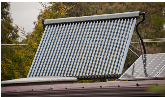
Evacuated tube solar collectors are more efficient than flat plate systems.
