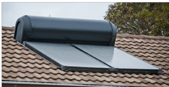
Roof mounted flat plate solar collectors and hot water tank.
