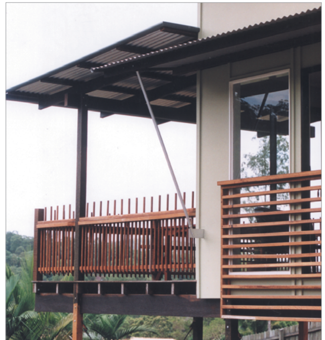
This adjustable shade screen can exclude low angle sun.
